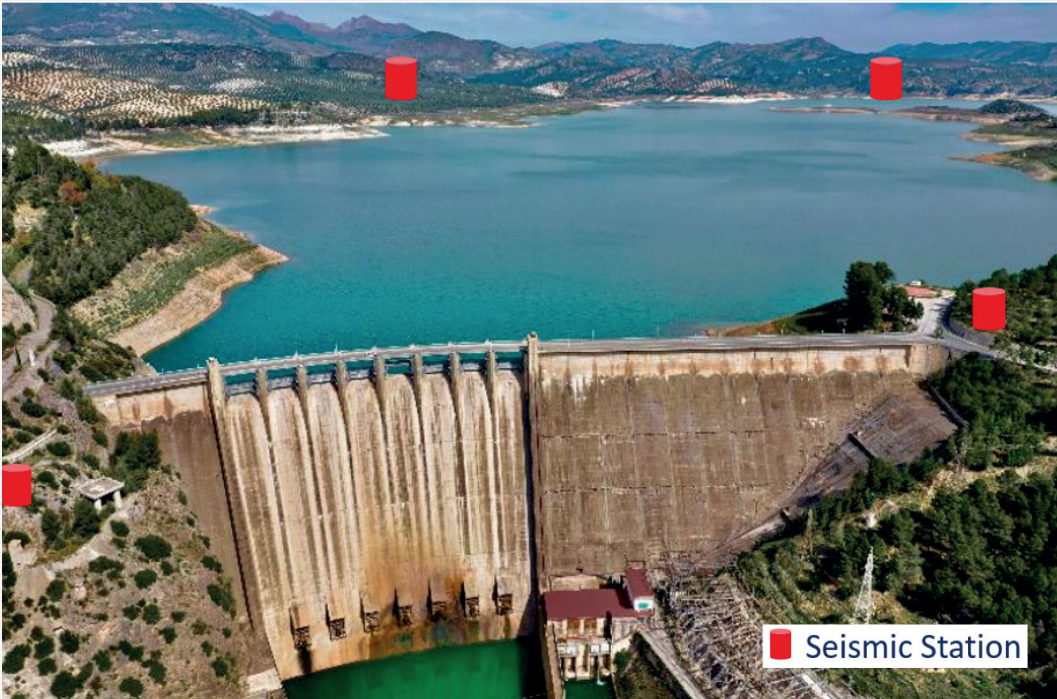
Figure: An example layout of seismic stations for KMIDam RIS.
