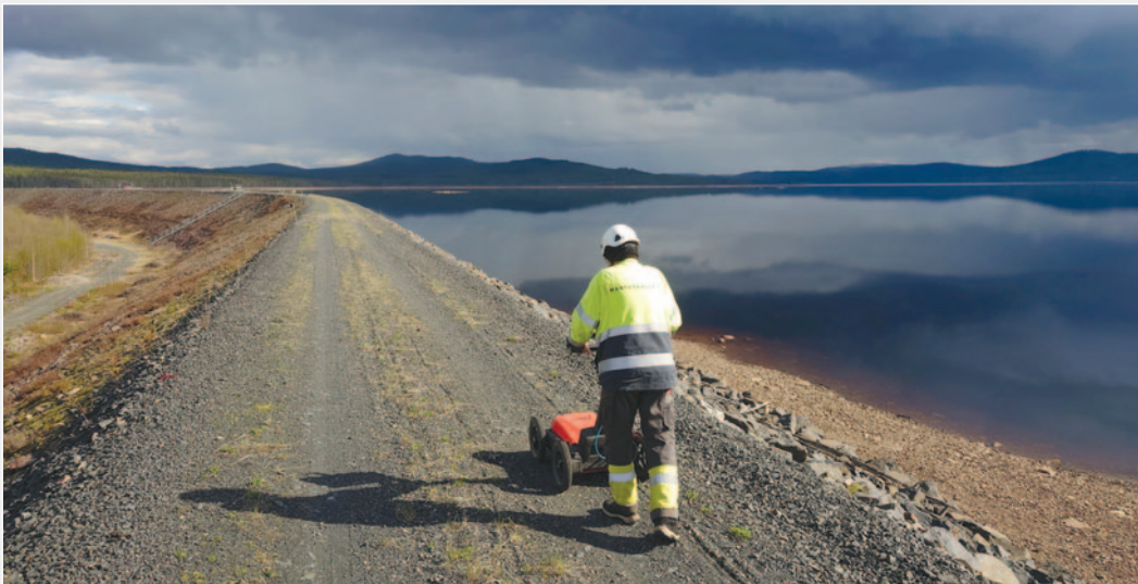
Inspecting an earthen dam.
