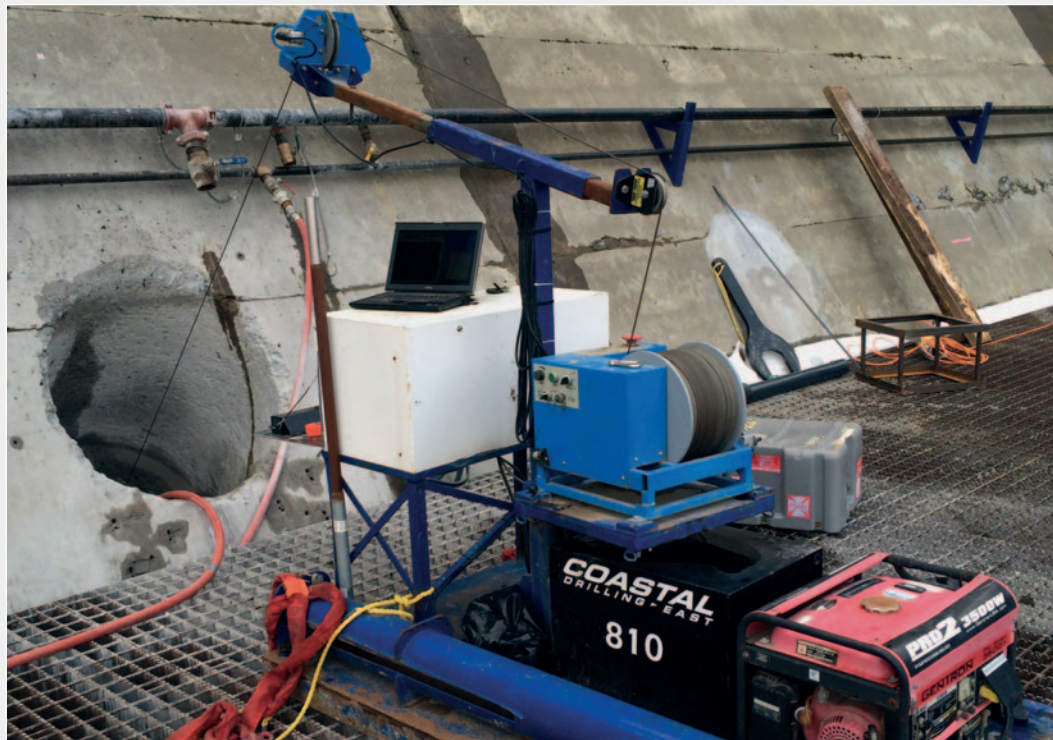
Robertson Geo 600m Winch in action for the Televiewer application at Bluestone Dam.
