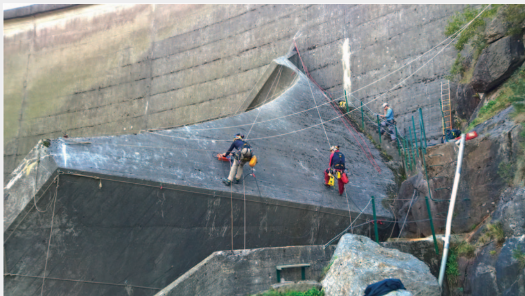
Inspection of dam reinforcement in Lapalisse, France.
