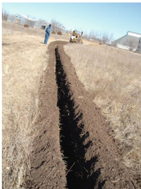
Fig. 24 Distributed strain sensor installation in a trench
