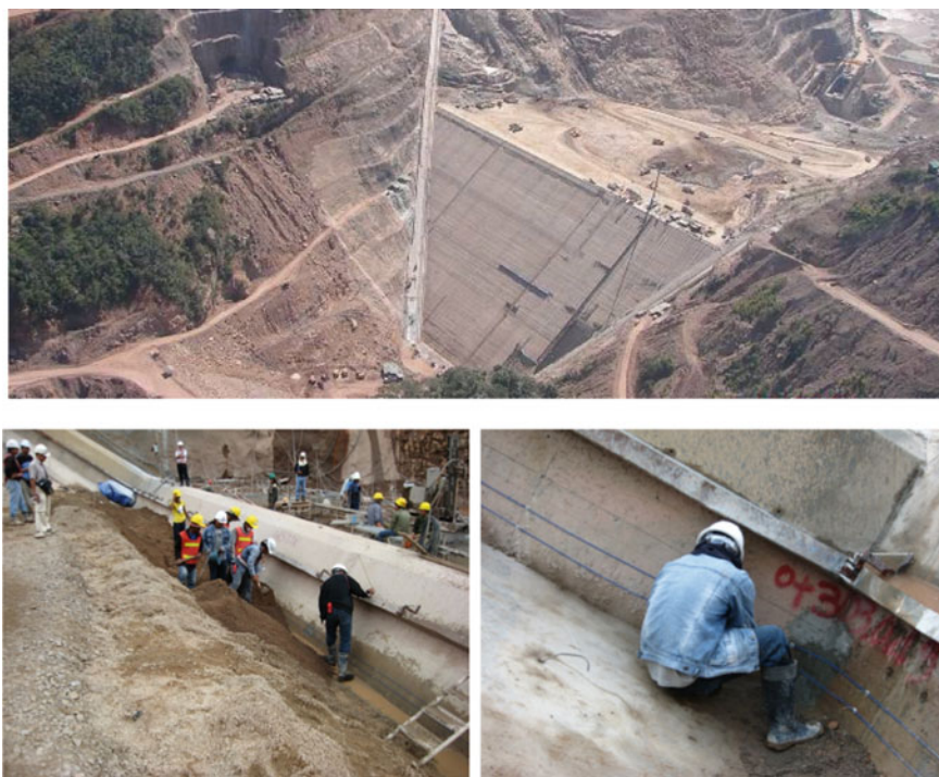
Fig. 13 Distributed temperature sensing cable installation along the plinth dam of the Nam Ngum Dam, Laos
