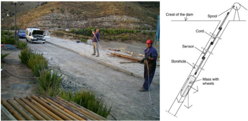
Fig. 28 Installation of long-gauge strain sensors in a borehole
