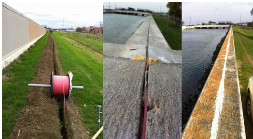
Fig. 17 Installation of distributed strain and temperature sensing cables in the levee foundations and on top of the I-wall and T-wall sections in New Orleans, Louisiana, USA
