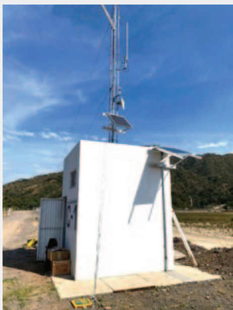
Exterior of iDAM seismic monitoring network station.
