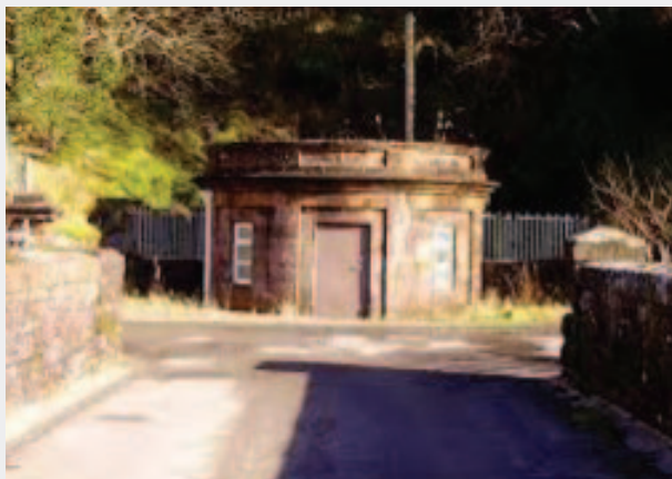
Talla Dam control room.
