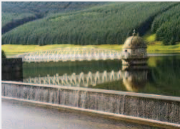
Talla Reservoir spillway and tower.
