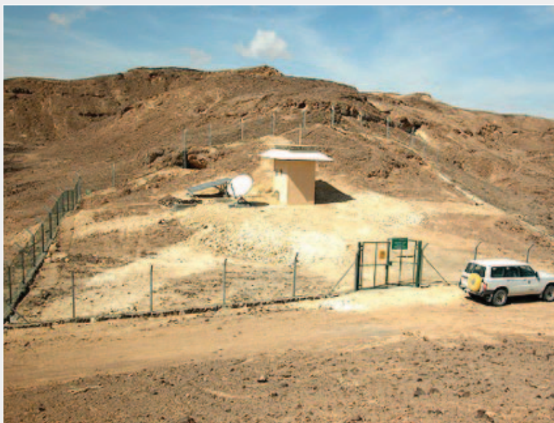
EMC network Aspen remote station.
